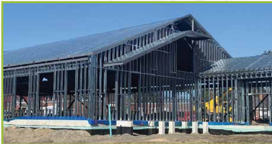
Northern Light CA Dean new hospital construction.
